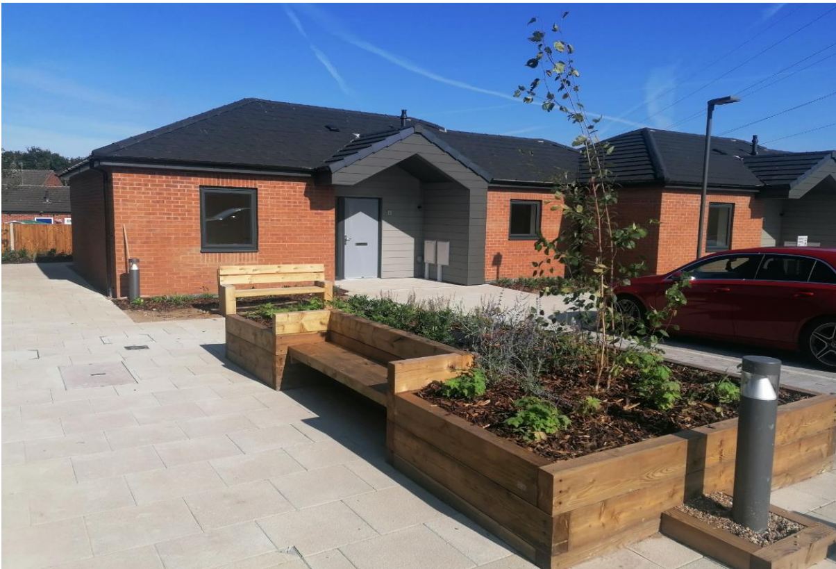
Two Bedroom Supported Bungalows at Broadleaves
